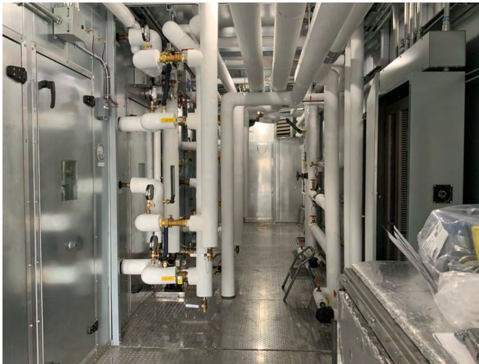
Figure 1: This photo shows the hot water and chilled water piping within the service vestibule of a semi-custom unit used on the Hackensack Meridian hybrid OR project. The piping and equipment within the service corridor was designed to allow the maintenance staff to walk within the unit and access all the components. Courtesy: Syska Hennessy
