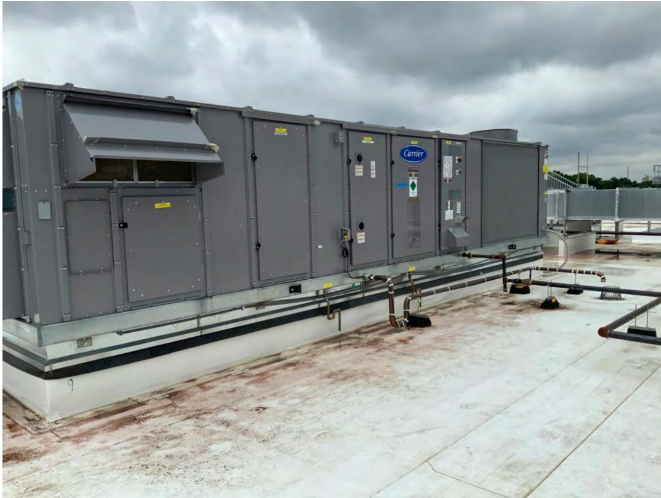
Figure 5: Shown is an example of a semi-custom unit used for a health care facility. The unit comprises supply and return fans, a direct expansion refrigerant cooling coil, gas heating, pre- and final air filters and an air-side economizer. Courtesy: Syska Hennessy
