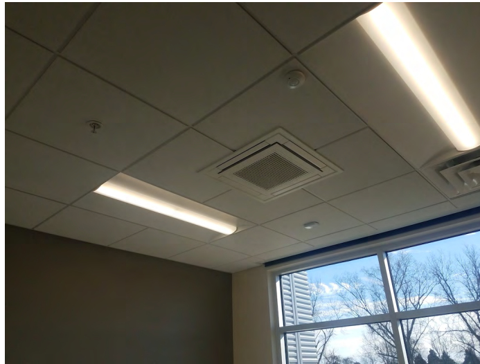
Figure 4: Delivering dedicated outdoor air directly to a space using traditional diffusers and grilles is common in chilled beam applications. Courtesy: Smith Seckman Reid Inc.
