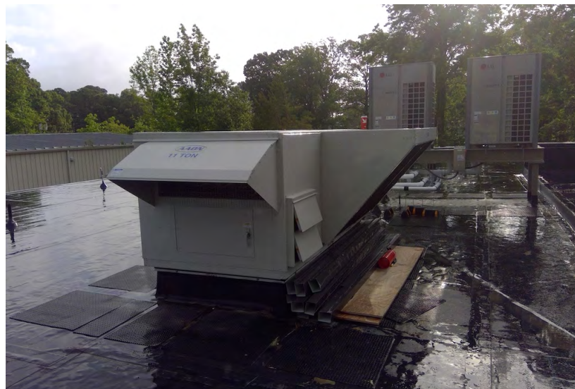
Figure 6: This 11-ton, roof-mounted, packaged dedicated outdoor air system is a heat pump that uses a separate variable refrigerant flow system to heat and cool individual spaces. Courtesy: Smith Seckman Reid Inc.
