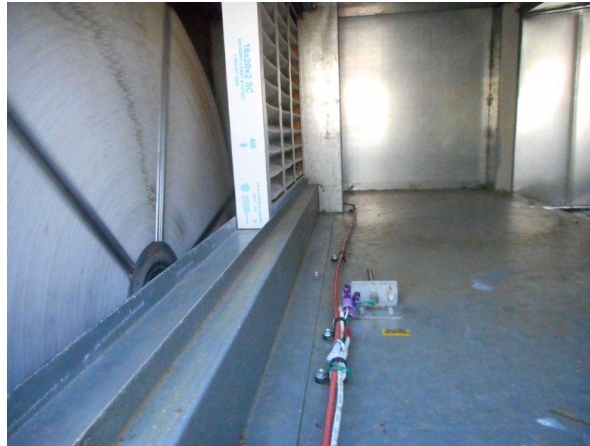
Figure 2: The status of an enthalpy wheel is key for energy efficiency considerations and temperature measurement. Courtesy: Smith Seckman Reid Inc.
