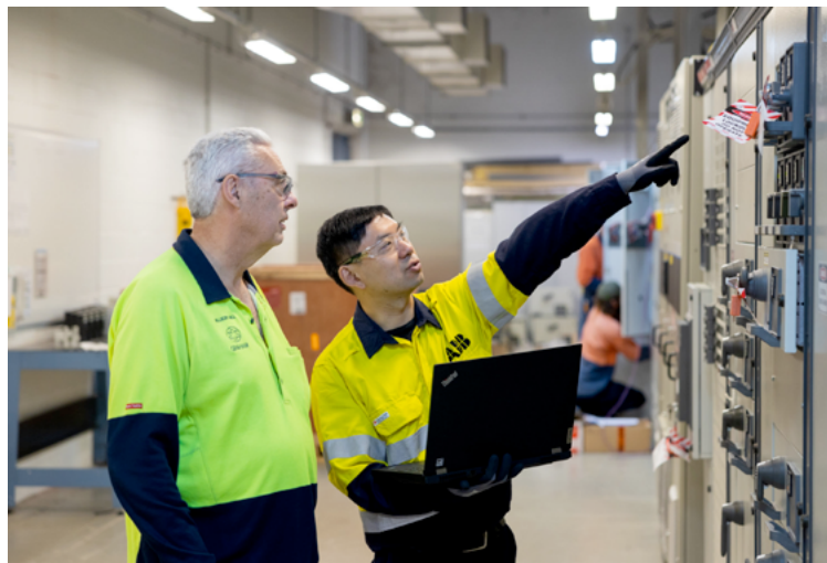
Figure 1: NFPA 70B assists equipment owners and maintenance teams in the development of electrical maintenance plans that deliver operational safety and optimal reliability while minimizing the operational cost of ownership. Courtesy: ABB Electrification, Service Division
