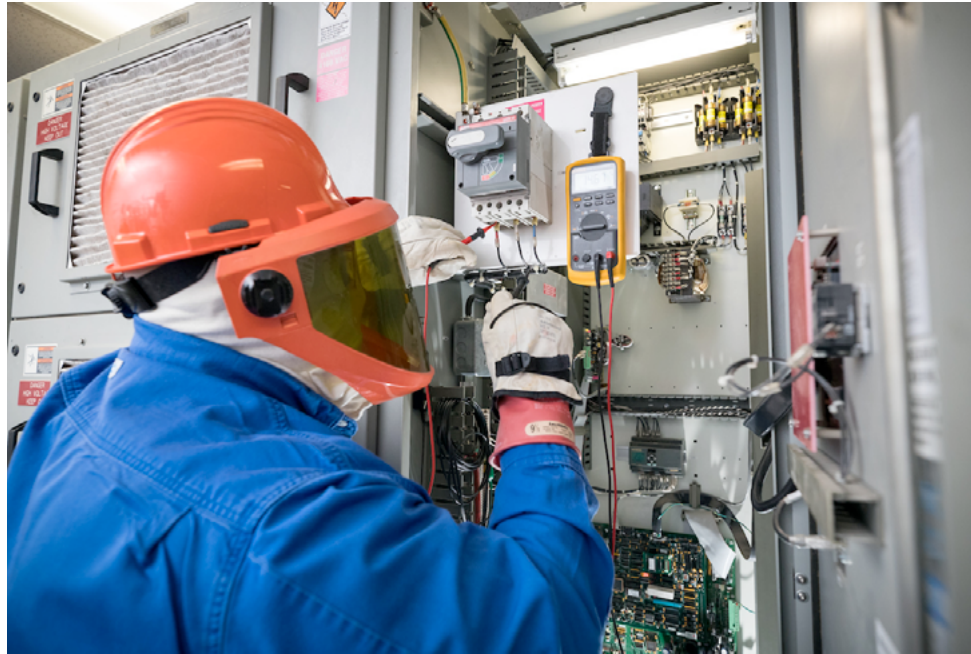
Figure 3: Proper PPE is a must when working on energized equipment. Courtesy: Shermco Industries
