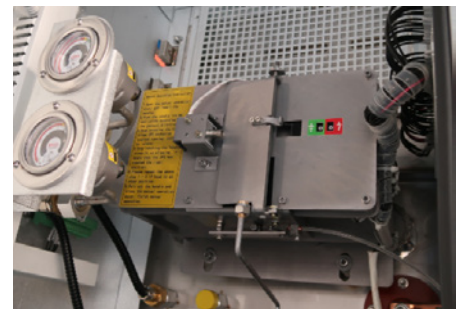
Interlocked three position disconnect switch for isolating and earthing with electric operation
